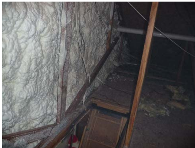
Figure A40. Floor cavity and knee wall after repair in garage attic
