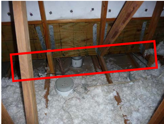
Figure A27. View of pathway from the garage (east) attic into a floor cavity, which results primarily from a dropped ceiling over the kitchen.
