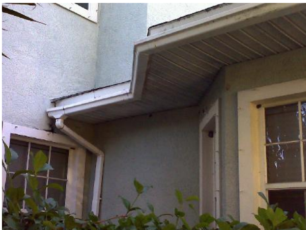
Figure 23. Photo of exterior west-facing wall
