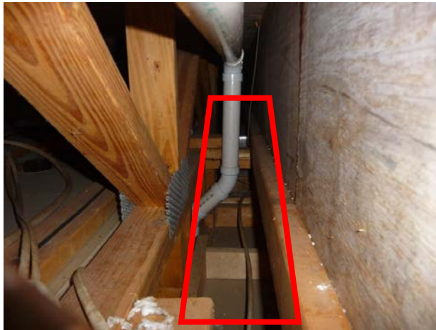
Figure A30. View of the inside floor cavity at corner leak in preceding figure. A large area of the floor cavity is effectively covered by well-placed plywood, but air circumvents this from under the dropped ceiling area at the red box.
