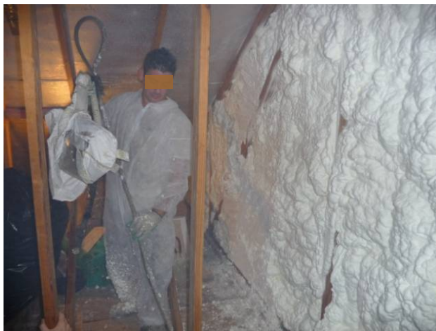
Figure 33. Foam insulation was used to seal the attic-to-floor cavity opening and insulate the knee wall above the floor cavity opening in Phase 1 House H16B.
