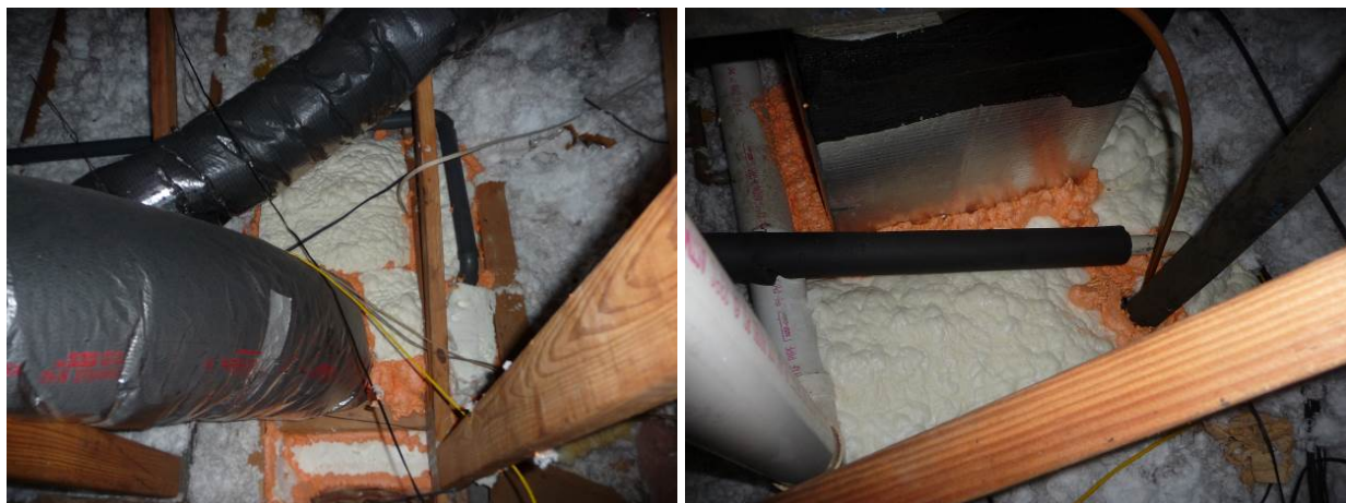
Figure A41. Vertical duct chase openings in second-story attic after sealing with foam
