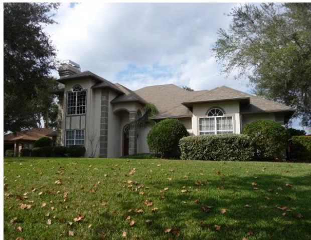
Figure A25. Front of House H39L faces southward. The garage attic is on the east side (right).
