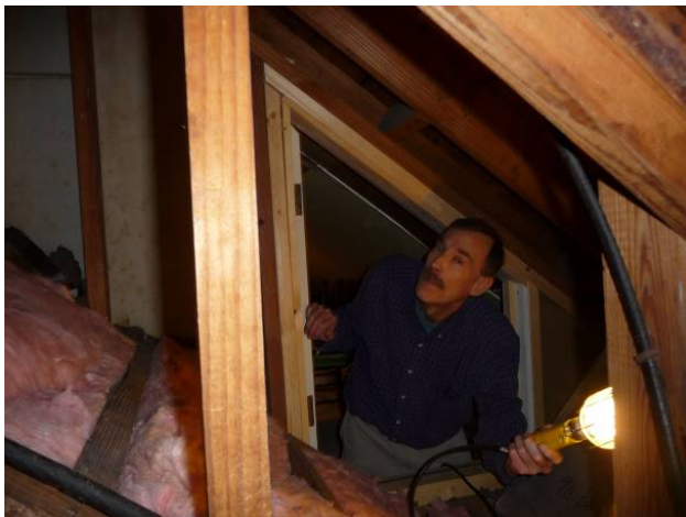
Figure 4. House H36M. Research team member performs a visual inspection in the attic space. Each accessible attic space is inspected to identify the presence and magnitude of wind washing characteristics.
