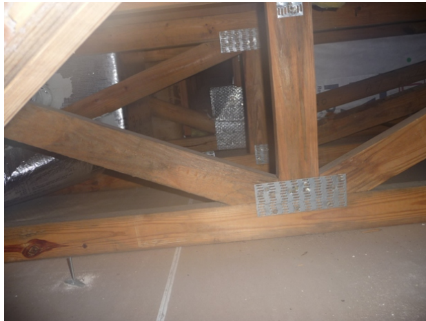
Figure A3. Looking from east attic space into open floor cavity (view toward the west)
