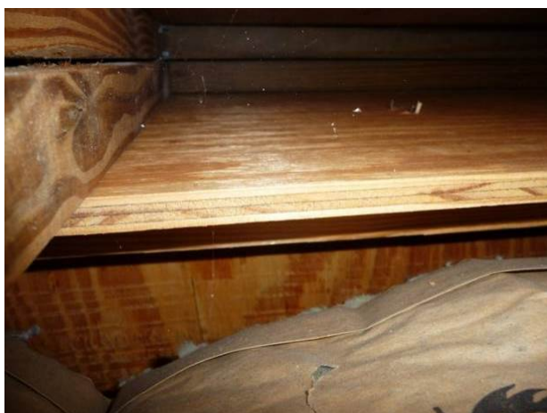
Figure A11. View looking up into a vacant wall cavity from within the east attic shows no insulation in this wall next to a walk-in closet.
