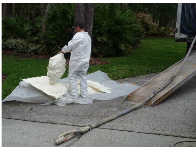
Figure A42. Foam plugs used to seal the second-story attic chase pathways were created outdoors, then easily carried up to the repair site.
