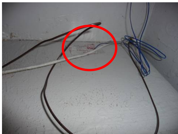
Figure 32. A thermocouple was inserted into the supply plenum (through the side wall of the plenum behind the foil tape) of the second-floor heat pump system to sample supply air temperature at House H39L.
