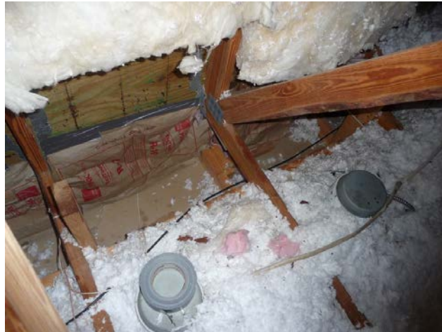
Figure A31. Sealing vertical plane of pathway with paper mechanically fastened and adhered to solid plywood above and adhered to the drywall ceiling below. Duct tape is not a lasting seal, but is used to reinforce the paper edge and provide temporary support during final placement.
