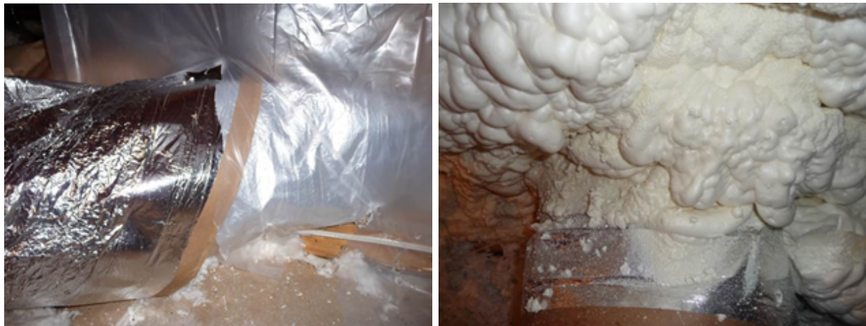
Figure A13. Photo on left was taken during the preparation to protect cold air supply duct with an insulating wrap having vapor barrier on outside. Photo on right is a view over top of duct after the wrap was carefully attached and foam was applied.
