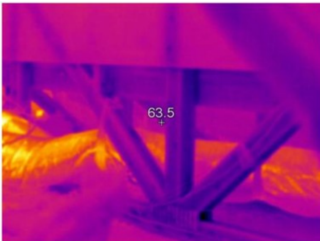
Figure 24. IR image of openings between the east attic and floor cavities near the second-floor bathroom
