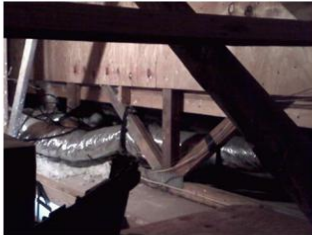
Figure 25. Photo of openings between the east attic and floor cavities near the second-floor bathroom
