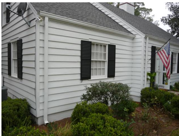
Figure A14. Front northwest corner of 1940s era House H36M. The west attic area is over the room on the northwest corner.
