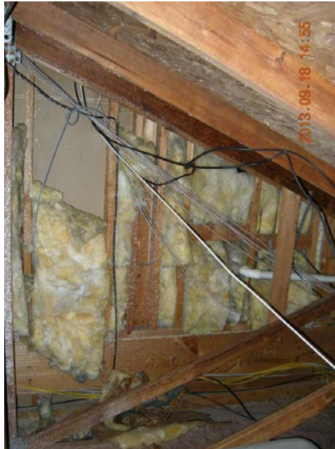
Figure A39. Garage knee wall with R-11 insulation in very poor condition. The irregular framing pattern and numerous wires make it more difficult to adequately insulate with fiberglass batts.
