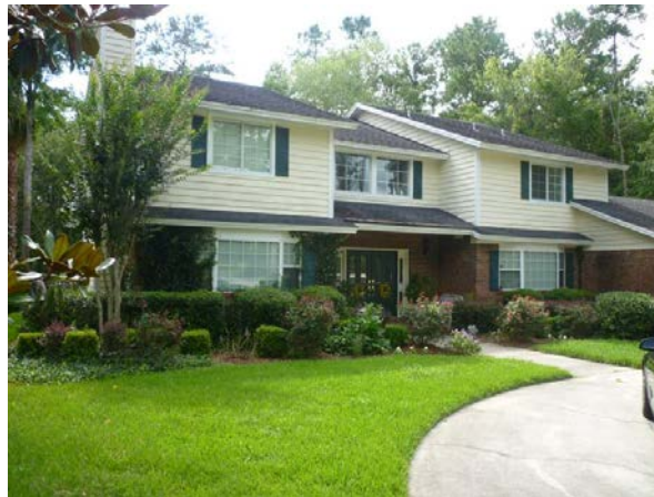
Figure A36. Front view of House H47W
