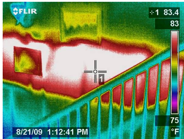
Figure 17. Summer IR image shows where hot attic air has penetrated into the floor cavity that lies behind the stairwell wall. The wall surface temperature at the floor cavity interface was 83°F compared to 77°–78°F room air temperature.
