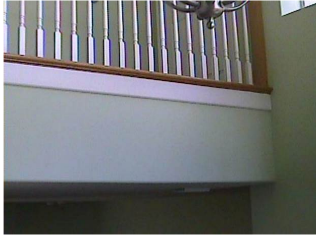
Figure A8. Photo of second-floor landing
