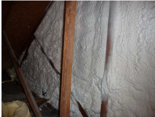
Figure A24. Finished view of foam sealed and insulated floor cavity and knee wall of House H37M
