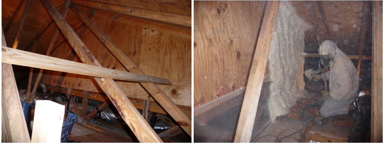
Figure A12. East side of floor cavity and knee wall before and during repair with spray LDF.
