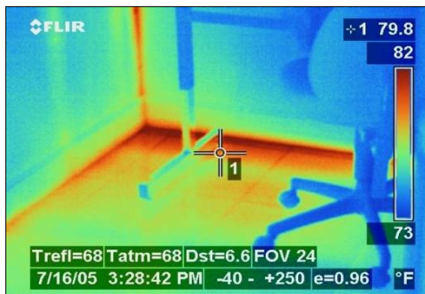
Figure 2. Elevated floor temperature results from hot attic air flowing through the floor cavity.
