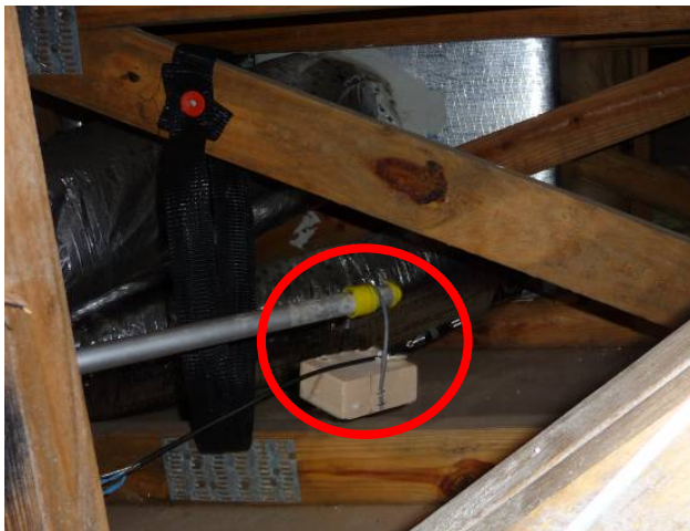
Figure 30. A telescoping pole was used with a portable mounting block to place a Vaisala temperature/RH probe inside the floor cavity at House H23K. Sensors were located away from ducts and duct leaks.
