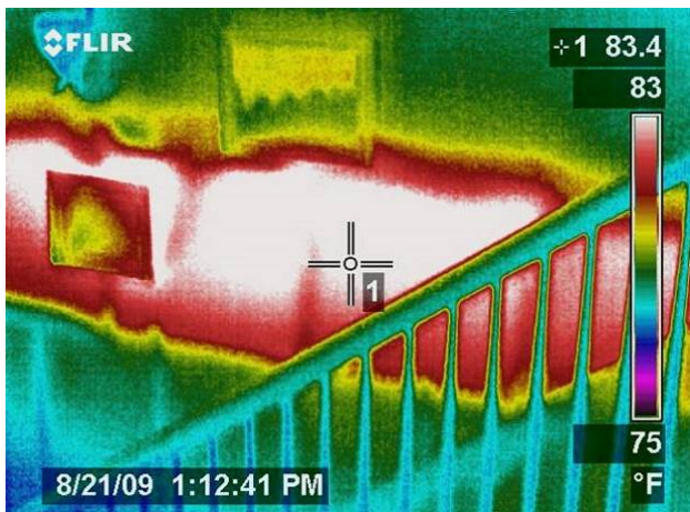
Figure A5. IR image shows where hot attic air has penetrated into the floor cavity that lies behind the stairwell wall.
