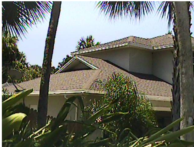
Figure A1. East and north sides of House H23K with garage attic adjacent to open floor cavities
