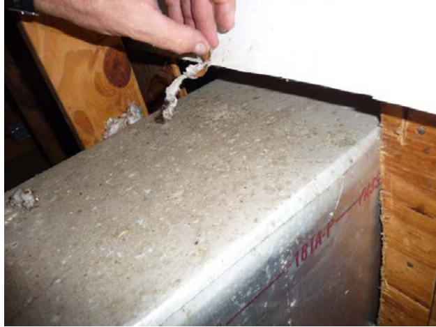
Figure A26. Air flows from floor cavity into west attic area pushing paper away from floor cavity leak toward the attic space. This leak is a complementary pathway to larger floor cavity leakage in the east attic.
