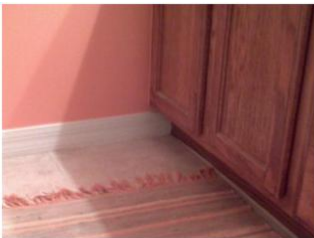
Figure 21. Photo of bathroom floor
