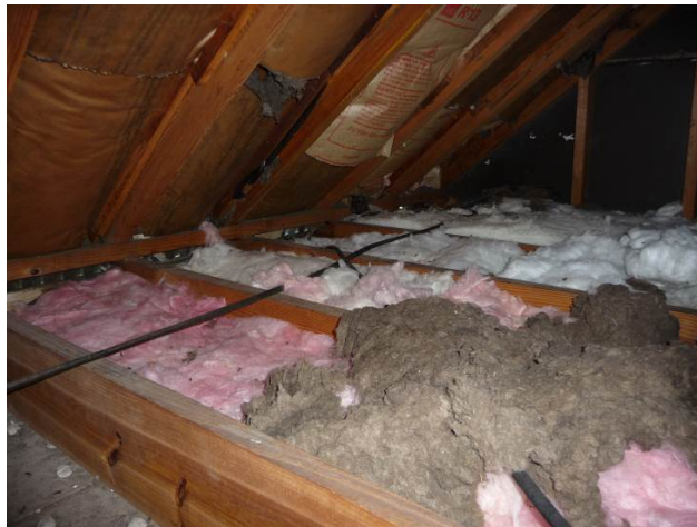
Figure A16. Pieces of old batt insulation, which have fallen from the roof deck above, can be seen in one area on the attic floor.
