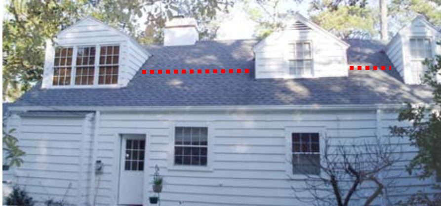
Figure A15. House H36M east back side where the shallow east attic is located. The vertical plane of the knee wall and floor cavity is approximately at the red dashed line.
