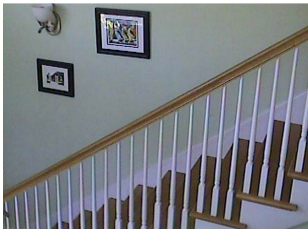
Figure A6. Stairwell where the wind washing thermal impacts is occurring
