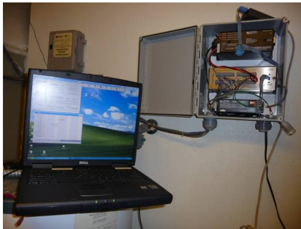
Figure 27. Installed data logger shown connected to sensor wires and to laptop at House H39L
