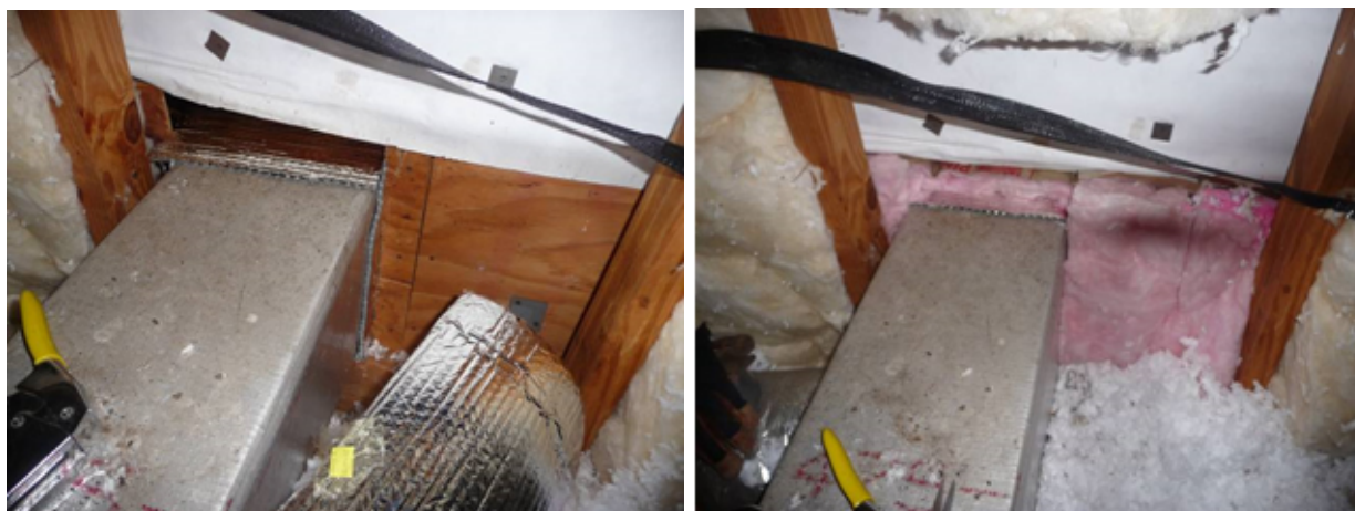
Figure A33. Repair in the west attic at duct penetration starts with application of a thin insulated vapor barrier placed against the cold supply duct. Then, batt insulation was placed against the vapor barrier.
