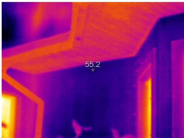
Figure 22. IR image of exterior west-facing wall. The soffit vent area is about 57.8°F.
