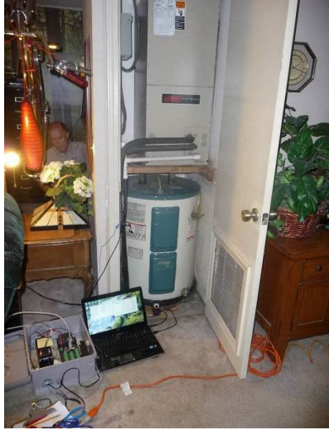
Figure A22. This closet operates as a return plenum (shown with door open during data acquisition system installation). A data logger can be seen on the floor next to the laptop.
