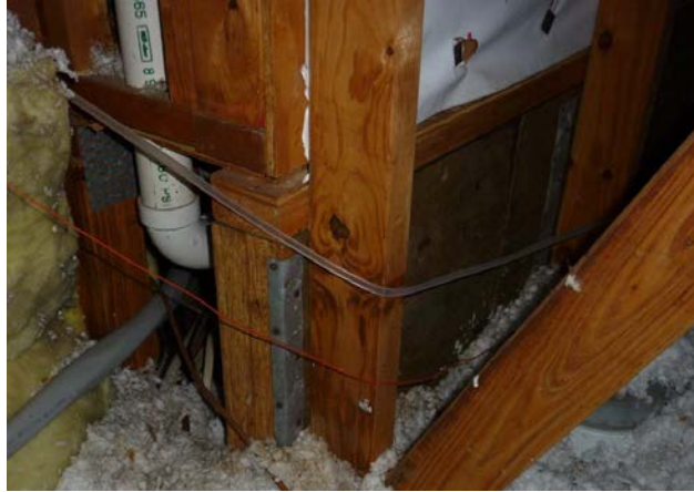
Figure A29. Corner of floor cavity with an air pathway around wire and plumbing penetration and a large area on the right side effectively blocked by plywood
