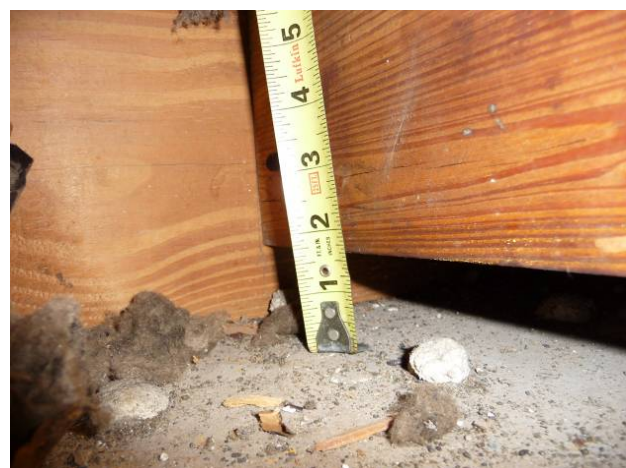
Figure 9. Most of the openings between the attic and floor cavities are blocked by frame members, leaving a 1- 5 / 8 -in. gap that occurs continuously. Pieces of original dirty insulation (R-11) have fallen from the roof deck above.
