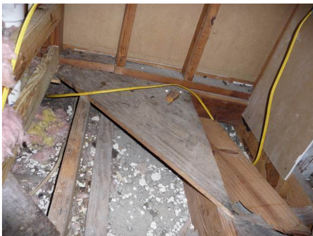
Figure 6. House H36M. View inside an east attic floor cavity section, with uninsulated knee wall area above. Complementary wind washing pathways are located at the other end of the floor cavity in the west attic.
