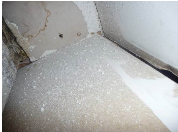
Figure A23. View of AHU closet ceiling. The closet, which operates at negative pressure because it is a return plenum, is very leaky to the second-story floor cavity as a result of unfinished drywall wall at the corner and large gaps in the ceiling. Some areas of air leakage were identified by squeezing a digital camera into tight areas between the AHU and the wall.
