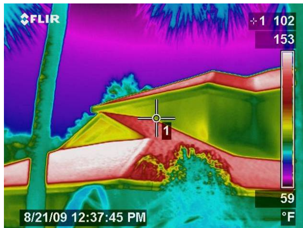
Figure A2. IR image of the house at midday after mostly sunny conditions all morning
