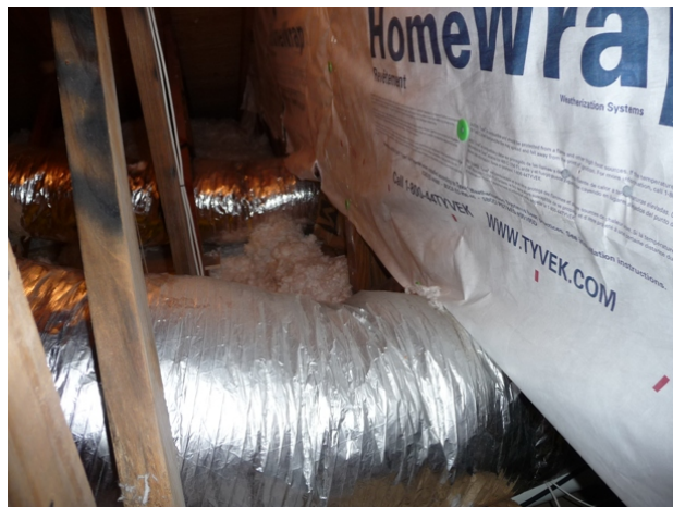
Figure A4. Looking at ducts passing from west attic into an open floor cavity
