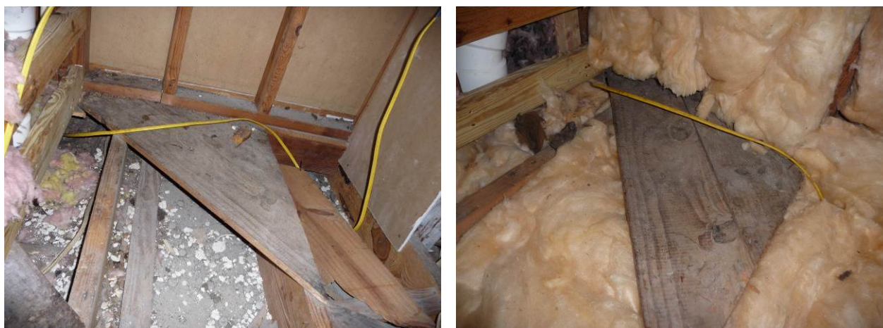
Figure A18. A section of unsealed and uninsulated floor cavity and knee wall in left photo and during repair with R-30 kraft-faced batt insulation installed in photo on the right.
