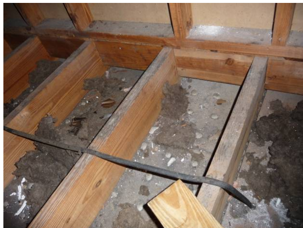
Figure 8. Most of the floor cavity openings from the west attic of House H36M are substantially blocked by frame members positioned between solid floor joists (see close-up in Figure 9).
