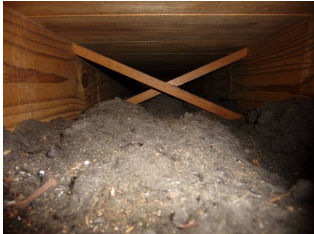
Figure 7. View inside one section of floor cavity from the east attic of House H36M. This floor cavity is wide open to the attic space.
