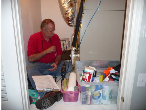
Figure 14. Preparing to measure the second-story AHU airflow rate at House H53 using a True Flow plate
