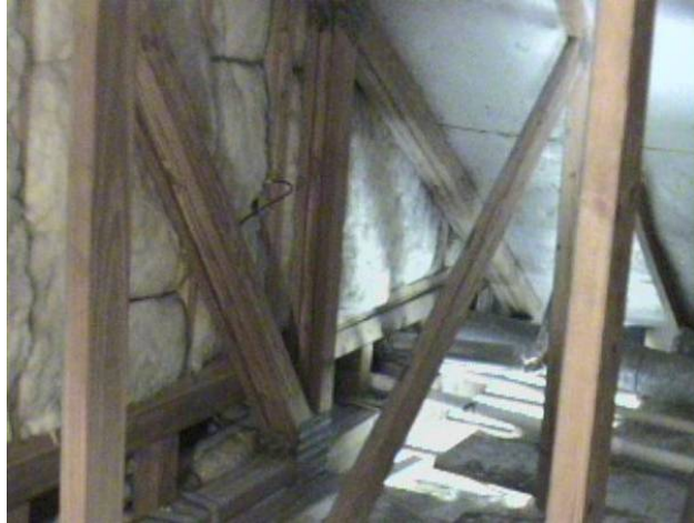
Figure 34. Floor cavity opening and knee wall can be seen in House H16B prior to foam insulation application.
