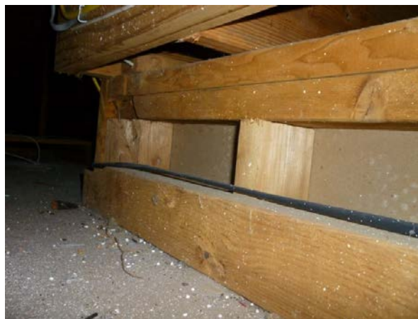
Figure A38. Second floor has a cantilever section inside the garage attic that resulted in a pathway about 3 in. wide by about 18 ft long.
