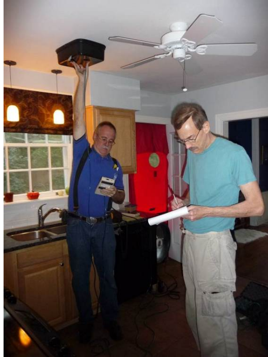
Figure 12. In House H36M, a Ppan test indicates both the magnitude and the general location of duct leaks with the air handling unit (AHU) off and the house depressurized to -50 Pa. The blower door fan in the background is used for both the house tightness and Ppan tests.
