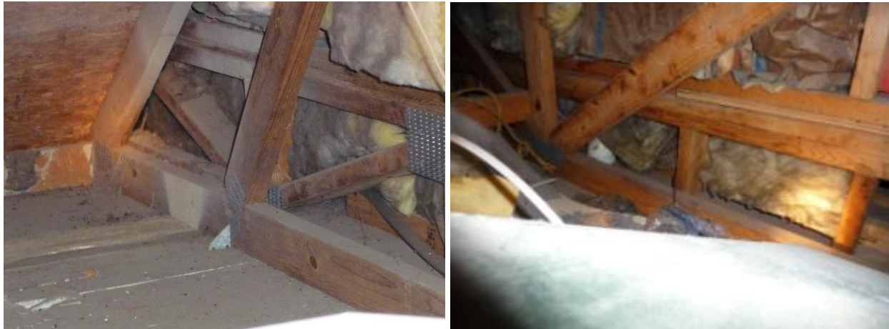
Figure A21. At left is a floor cavity section where existing batts do not seal the space. At right is another section with compressions and voids in the batt.
