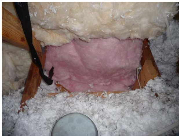
Figure A32. Section of completed repair with R-19 batt insulation fiberglass side out placed against the initial section of insulation in the previous figure. This is done to provide code-required fire ignition protection of the paper facing.
