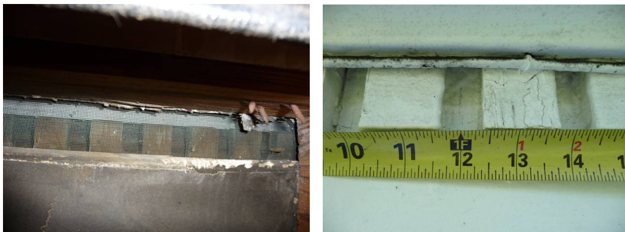
Figure A17. Dentil style attic venting viewed from inside attic and from outdoors. Venting is located along both east and west attic floor perimeters and has an insect screen on the attic side.
