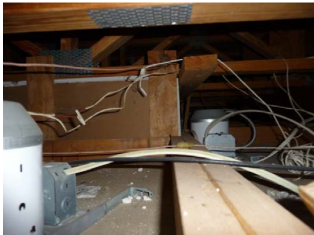
Figure A28. View from garage attic into the dropped kitchen ceiling with floor cavity above
