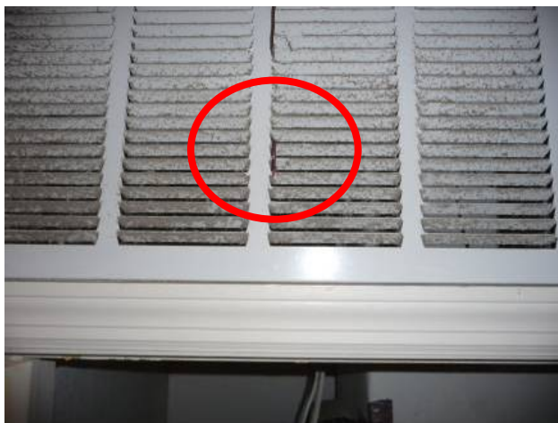
Figure 31. A copper-constantan (type T) thermocouple was used to sample return air temperature on the second floor of House H39L.
