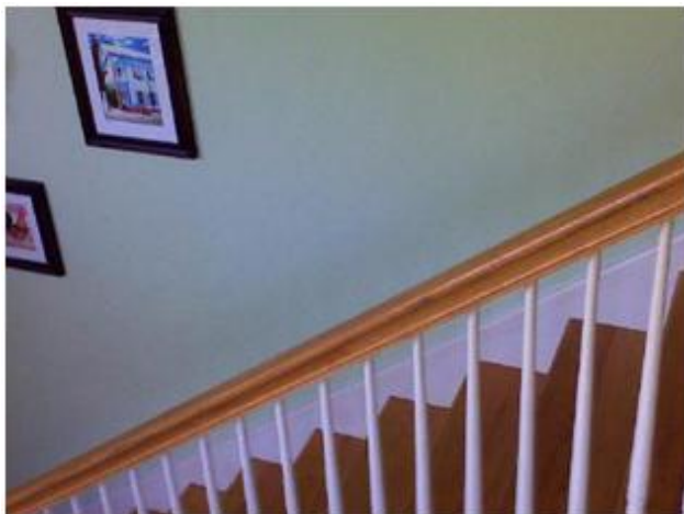
Figure 19. Stairwell where the thermal anomalies occurred
