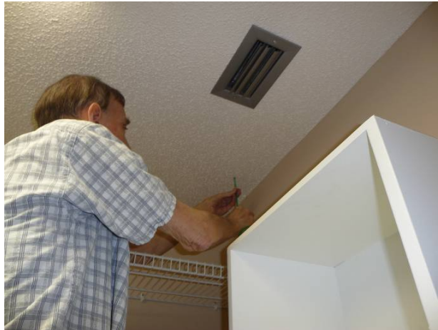
Figure 15. Floor cavity air pressure is measured by placing a tube into the floor cavity through a small drilled hole, with homeowner approval, at House H52.
