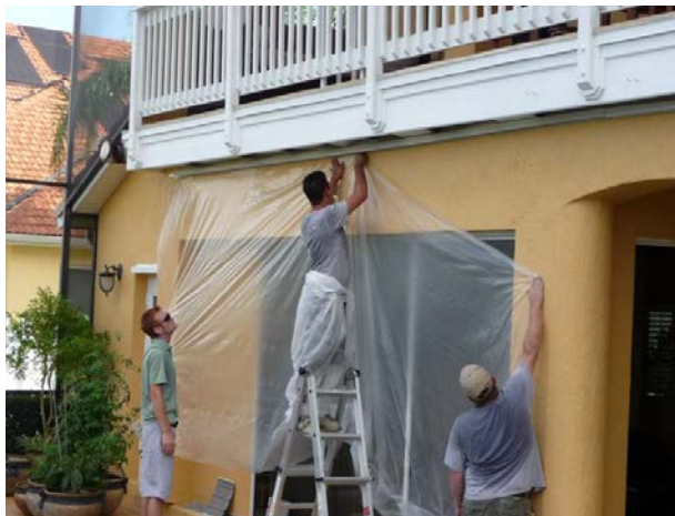
Figure 36. Exterior wall and window area was protected from potential overspray of foam applied within the soffit area above
