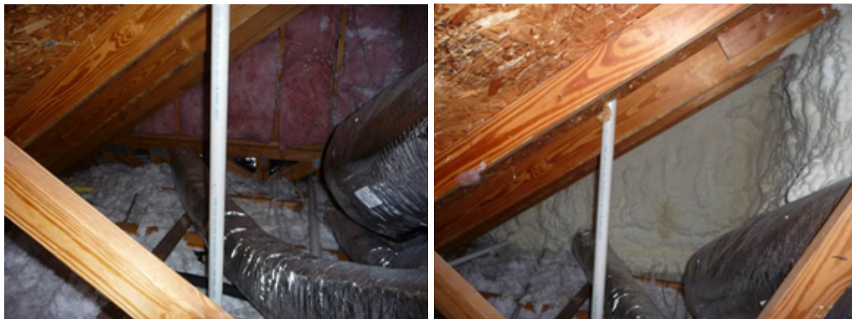
Figure A35. East side of floor cavity and knee wall before and after repair
