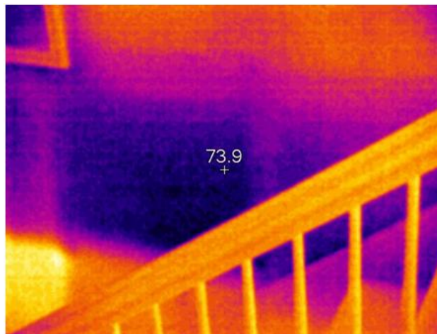
Figure 18. Winter IR image shows where cold outdoor air has penetrated into the floor cavity that lies behind the stairwell wall. The wall surface temperature at the floor cavity interface was 73.9°F, about 1.5°F colder than the room air temperature. Overnight low outdoor temperature was about 44°F several hours prior to the image with calm wind conditions.
