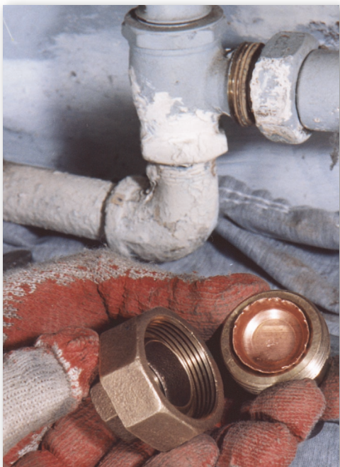
How a radiator inlet orifice fits between the curved faces of a union. This orifice is blank, that is, the hole is not drilled yet.
