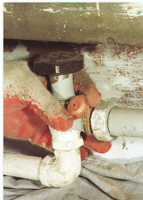
Radiator inlet orifice with the hole drilled.
