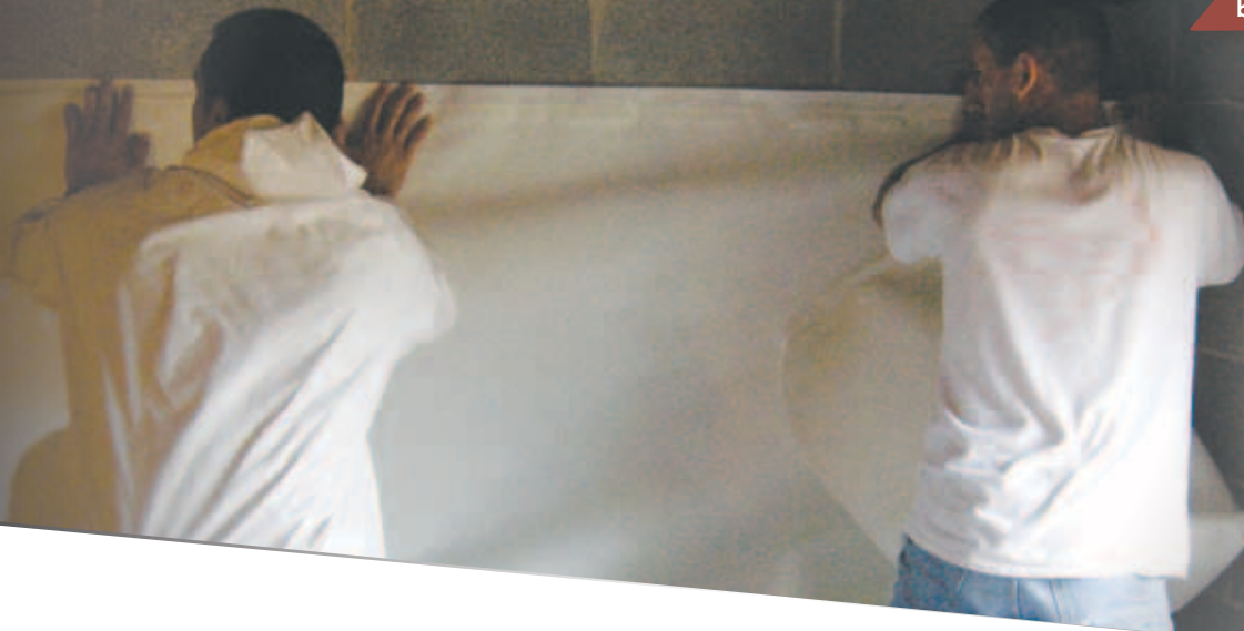
Applying wall liner with adhesive.
