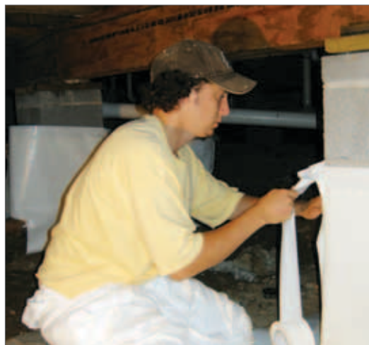
Preparing a post.
