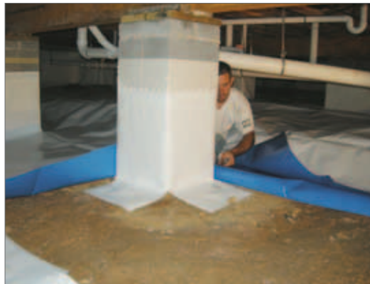
Laying a floor.
