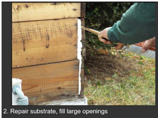
Figure 4. Installation Step 2
