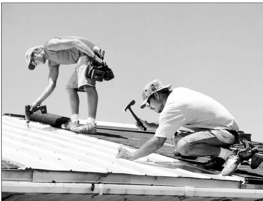
Roofers install unfinished metal roofing on the Flexible Roof Facility.
