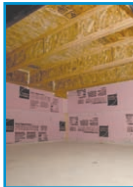
A well-sealed and insulated conditioned crawl space in a new home.
