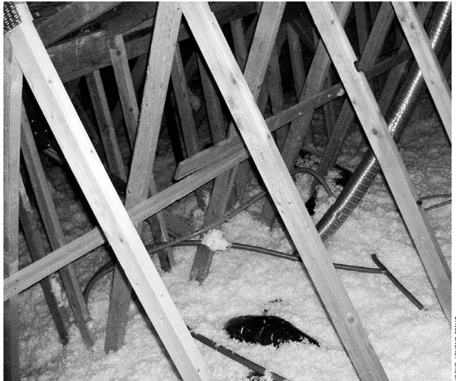
DAVIS ENERGY GROUP
