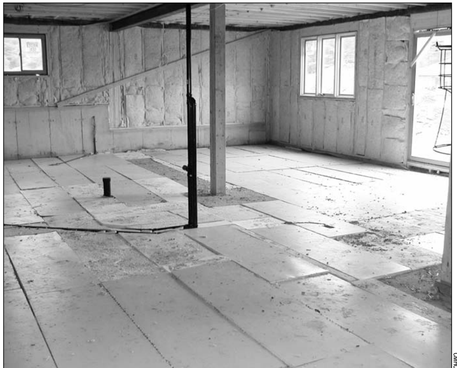
The Canada Mortgage and Housing Corporation tested the performance of foil bubble pack and other subslab insulations.
