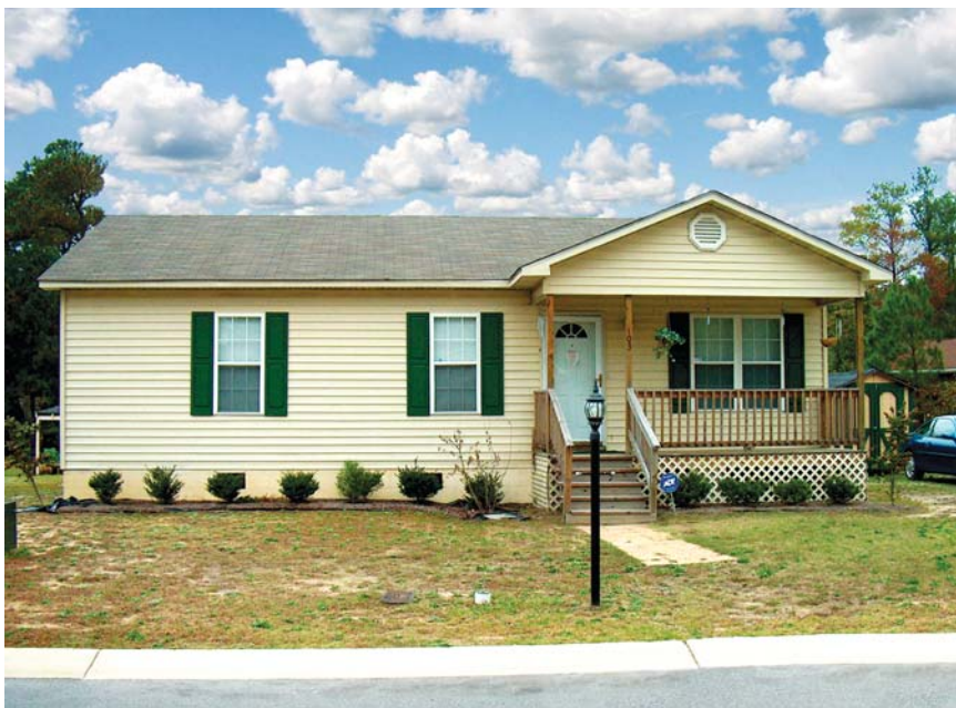
Closed crawlspaces represent both a new business opportunity and a risk management tool for many different stakeholders in the construction industry.
