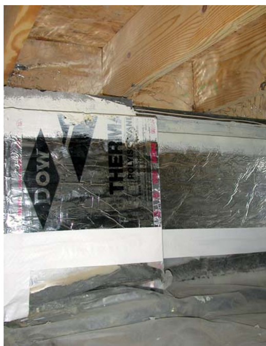
This wall-insulated crawlspace uses 2-inch-thick foil-faced polyisocyanurate insulation. The foam plugs in the band could be replaced by sections of batt insulation. A termite inspection gap is visible at the top of the wall insulation.
