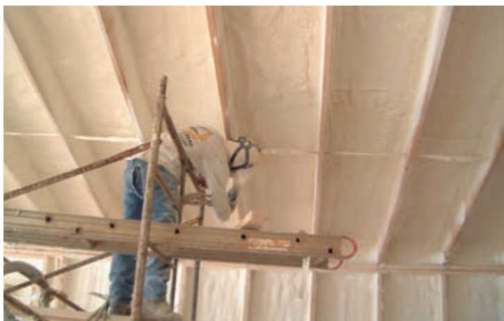
A technician applies closed cell foam to an unvented attic assembly.
