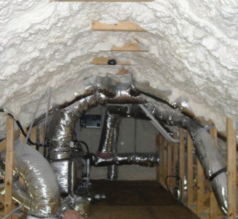
Attic roof deck with open cell foam applied. Notice all mechanicals are now located in the conditioned space.
