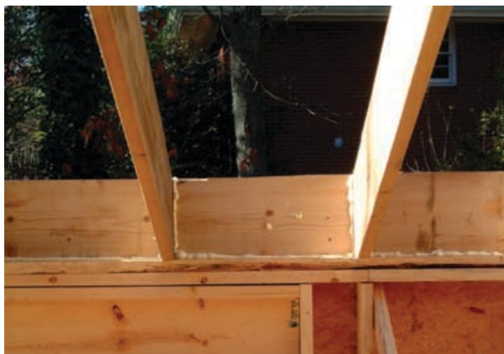
Blocking has been applied between rafters to ensure foam does not fill the soffits.
