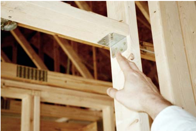
Photograph 5: Interior Wall Framing - Also framed on 24-inch centers. But these ones are 2x4's. And almost all of them are not load bearing so the connections are pretty much non-structural.
