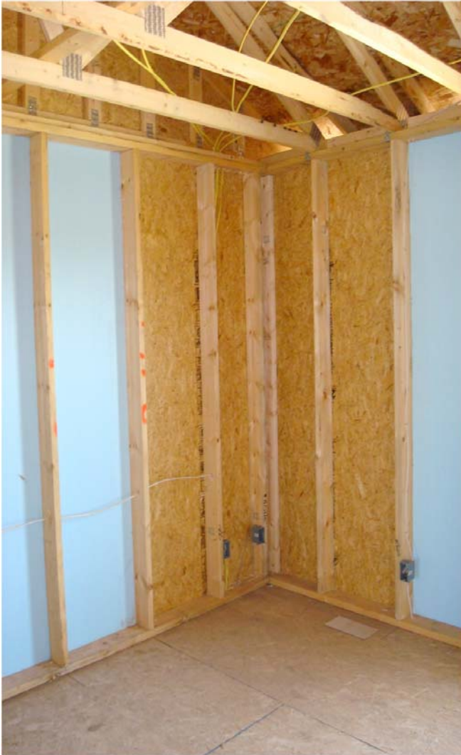
Photograph 7: OSB Braced Wall Panels - Insulating sheathing provides no “racking resistance” or “shear” properties. For that we need OSB or plywood braced wall panels – and most builders build them into corners.
