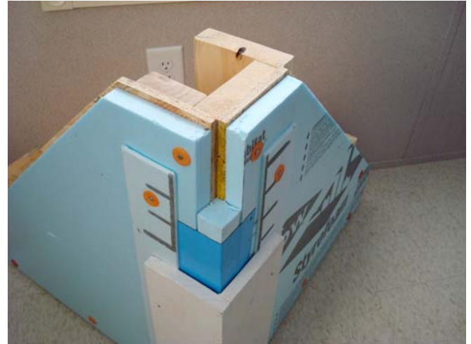
Photograph 8: Corner Framing With OSB and Insulating Sheathing – Note that the foam sheathing is reduced over the OSB shear panel so that the thickness of both sheathing layers line up with the thickness of the sheathing in the field of the wall. Also, note the spacer strip between the cladding and the exterior face of the insulating sheathing to provide back ventilation and drainage of the cladding layer and trim.
