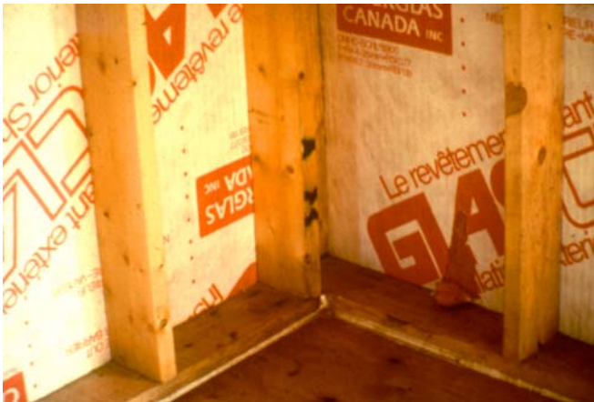
Photograph 3: Corner Framing - My first advanced frame building in 1982 using a two-stud corner.
