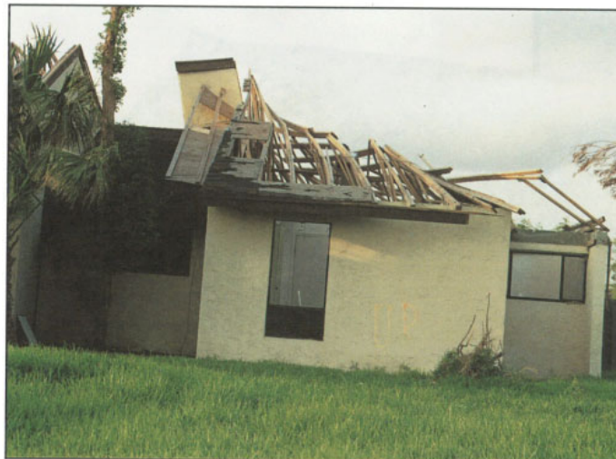
Figure 2. This roof structure failed during a hurricane due to inadequate bracing of the gable end trusses. (Source: FEMA, Building Performance: Hurricane Andrew in Florida, https://www.fema.gov/media-library-data/20130726-1611-20490-8788/fia22_sec2.pdf )
