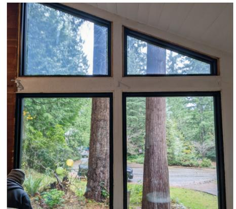
The new aluminum-clad-wood-framed windows have three panes of glass and low-emissivity coatings to resist heat transfer and to almost completely eliminate condensation risks.
