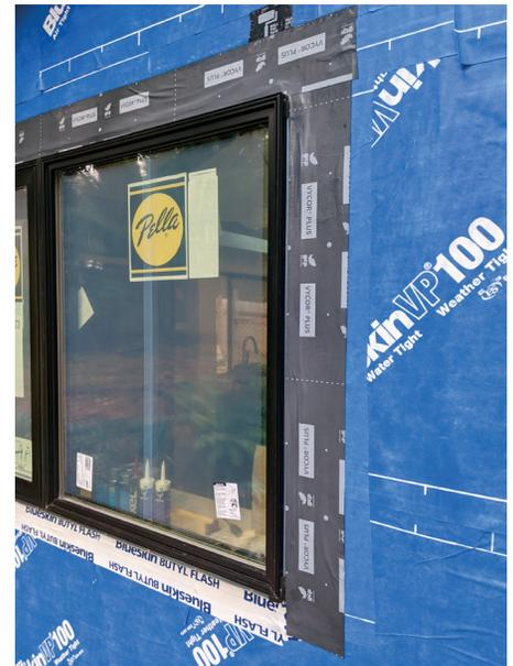
The installation of new windows provided the opportunity to wrap the rough opening with the self-adhered water-resistant membrane, to install flexible pan flashing on the window sill, and to properly integrate head and jamb flashing with the window flanges.
