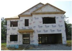
The XPS rigid foam sheathing is taped at the seams and covered with house wrap to provide a drainage, air barrier, and thermal barrier.
