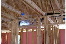
(Top) The walls use advanced framing with 2x6 studs at 24 inches on center and XPS rigid foam sheathing on exterior walls instead of OSB.
