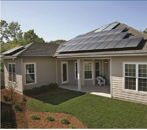
Tommy Williams Homes' first zero energy home was completed in January 2010 and had a tested HERS score of -2.
