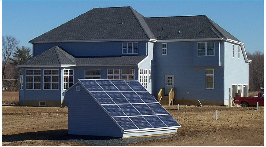
Tindall Homes installed their optional grid-tied solar photovoltaic systems on backyard garden sheds, situated for maximum solar gain. Wiring for the systems runs underground from the shed to the home's basement.
