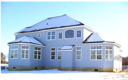
Insulated precast concrete foundation walls, spray foam-filled frame walls, and R-49 of attic insulation keep the Tindall homes in Columbus, New Jersey, warm in winter and cool in summer.
