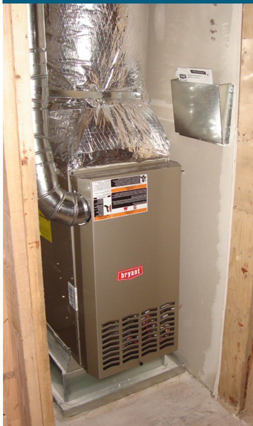
Building America recommended that Quadrant put the furnace and ducts in conditioned space to increase energy savings.
