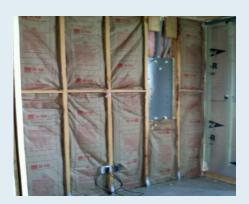
In many cases a properly installed thermal barrier can be compromised by holes or gaps in the air barrier. One approach to ensure the integrity of the air and thermal barrier is to delegate responsibility to one person to verify that air sealing is complete. While some builders may require electrical and plumbing teams to fill their own holes, this project found it effective to have one person follow these teams and ensure that all holes were properly sealed.
