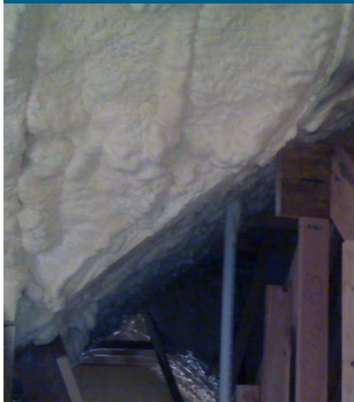
Unvented attics insulated with R-30 low-density spray foam provide a semi-conditioned space for the high-efficiency heat pump and ducts.
