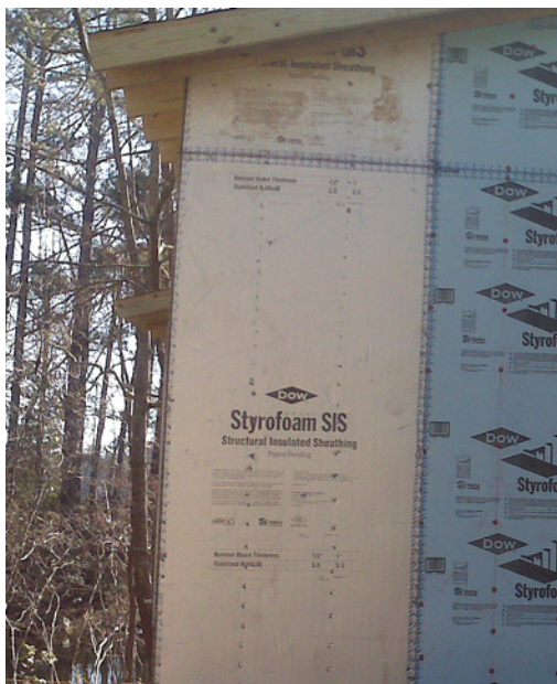
Framing is covered with XPS foam structural insulated sheathing instead of OSB. The foam sheathing provides R-3 of insulation and protection against moisture. The wall cavities are filled with an additional R-13 low-density spray foam insulation, which provides air sealing as well as insulation.
