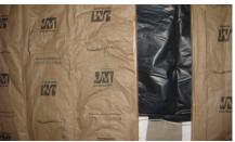
(*left*) In the crawlspace, R-30 fiberglass batts were installed between the 2x10 floor joists. The joists were then covered with 1 inch of expanded polystyrene (EPS) rigid foam board that was taped at the seams to provide a continuous air barrier and flashed at the edges to protect against rodents. The crawlspace floor was covered with a 6-mil visquene vapor barrier.
