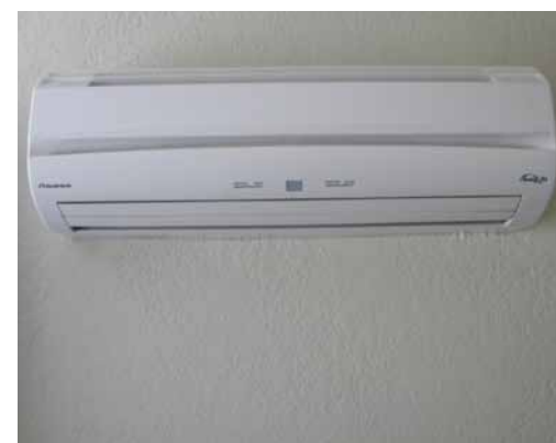
The home has never had a heating system. Building America researchers recommend installing a ductless, mini-split heat pump that will bring a year-round improvement in comfort. Wall-mounted units like this one will provide heating and cooling.
