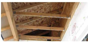
When the wall connecting the porch to the house is properly blocked and air sealed with OSB, dry wall, or rigid foam, a significant source of air and heat loss is removed.
