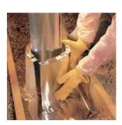
You can make a sheet metal or gypsum board dam to keep insulation from touching hot metal or masonry chimneys and flues (Source: EPA 2008a).
