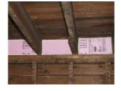
These floor joist bays have been properly air sealed with caulked rigid foam insulation.
