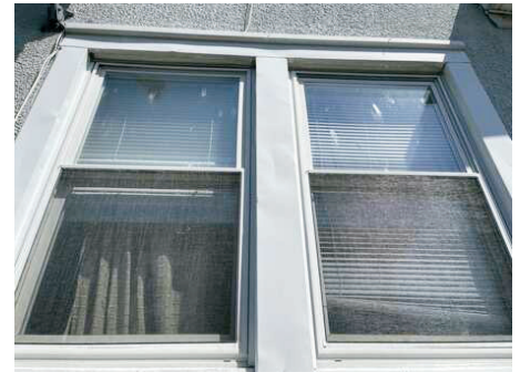
The deep frames of the existing windows would easily accommodate exterior low-e storm windows, which would help reduce both air leakage and heat transfer for lower energy bills and increased comfort along the exterior walls in the home. The low-emissivity coatings on the storm windows offer protection against both winter heat loss and summer heat gain for year-round benefits. Operable single-hung storm window models are available so the homeowner would not have to sacrifice the ability to open the windows once the storm windows were installed.
