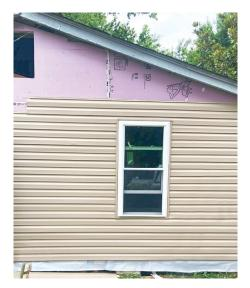
New vinyl siding was installed over the windows which were installed over new house wrap and 1 inch of rigid EPS.
