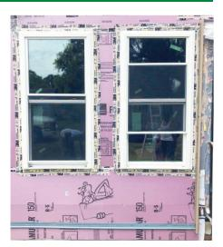
The original windows, an assortment of single- and double-pane metal- and woodframed windows were in bad shape. All were replaced with triple-pane vinylframed windows for energy efficiency and sound abatement. Note, at the bottom of the window, pan flashing is typically installed beneath the sill but tape is not installed over the sill flange.
