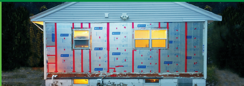
This 1946 kit home in Kalamazoo got new exterior foil-faced polyisocyanurate insulation and interior storm windows as part of a re-siding retrofit. The new insulation covers the walls but not the gable ends of the vented attic.
