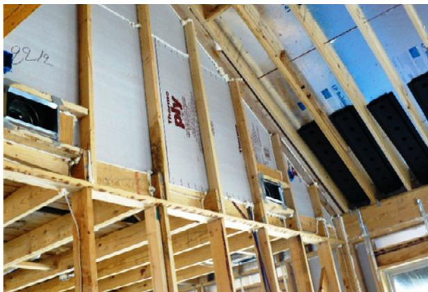
Advanced framing, which includes aligning all framing elements from the roof to sill plate, saves lumber. The savings more than offset the cost of additional insulation. The roof sheathing is lined with a radiant barrier to reduce solar heat gain for additional energy savings.
