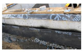
New Tradition Homes employs best practice recommendations for moisture management, including extensive site grading, below-grade drainage systems, damp proofing of exterior walls, contoured housewrap, gasketing of wall penetrations, and a waterproof gasket under the sill plate.
