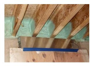
Building America research showed minimal insulation R value difference between spray foaming the entire opaque surface of a wall and spray foaming only areas known for leaks. The team used this "critical seal" approach for air sealing and cost savings at basement and second floor rim joists.
