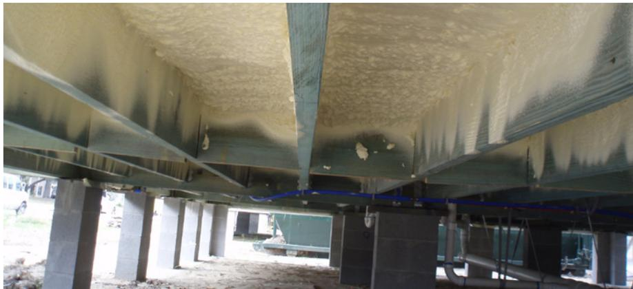
High-density closed-cell spray foam was sprayed between the 2x10 floor joists, in the 2x6 stud wall cavities, and along the underside of the roof decking to air seal and insulate. It also glues the components together to help the homes better withstand hurricane-force winds. All lumber is borate pressure-treated to resist rot and wall cavities are treated with an in-wall pest defense product.
