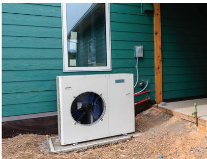
The split-system air-to-water heat pump provides efficient space and water heating and keeps the fan noise outside.
