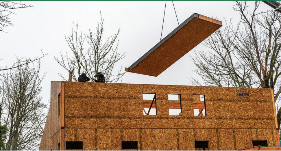
TC Legend Homes builds all its homes with SIP roofs and walls and ICF foundations. Clifton likes SIPs for their exceptional thermal performance with no thermal bridging and very little air leakage, racking resistance to earthquakes and high winds, minimal waste, and simplicity of construction. It takes just a small crew and a crane to put the homes together.
