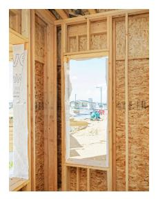
Advanced framing features include double walls with 2x4s at 24 inch on center, 2-stud corners, and right-sized window headers.
