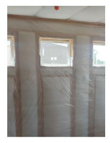
Garbett packed R-23 of blown fiberglass into the advanced-framed 2x6 walls and blew another 15 inches (R-60) into the vented attic.
