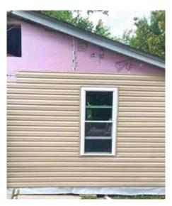
New vinyl siding was installed over the windows which were installed over new house wrap and 1 inch of rigid EPS.
