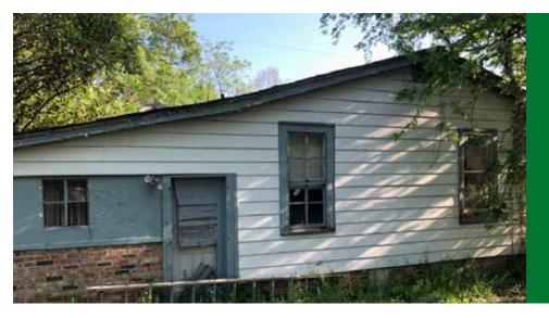
The home's original single-pane metal or wood-framed windows were in poor shape. Some were cracked, several were water damaged. All of the windows were replaced with triple-pane windows. Although the hot-humid climate of Jackson may not warrant high R-value windows for energy savings alone, the home's location near an active railroad line meant the sound-dampening effects of the triple-pane windows would be greatly appreciated.
