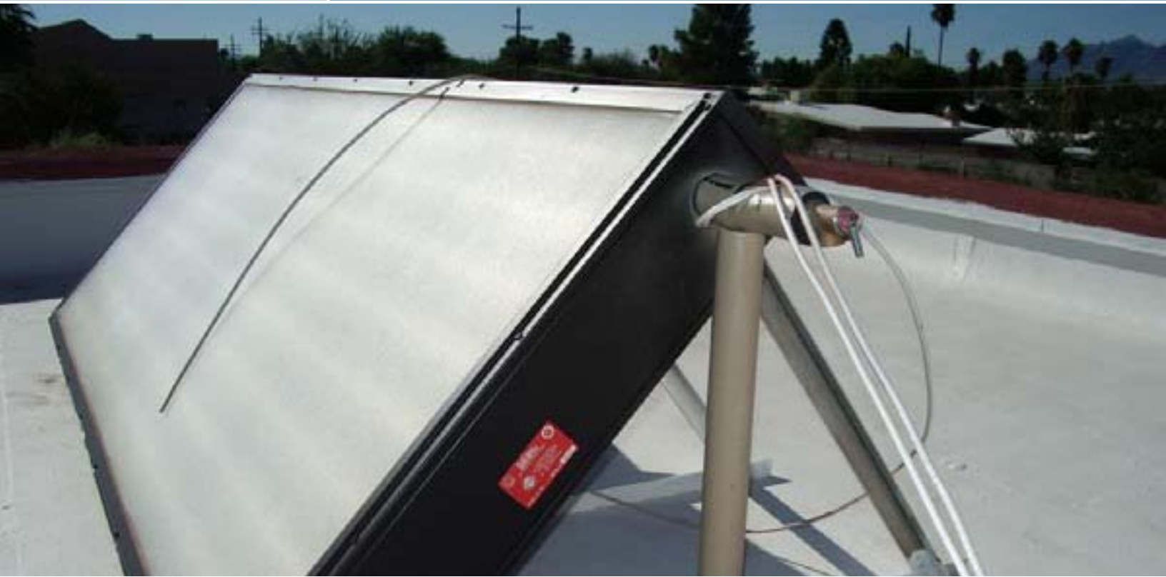
A Sun Earth Copperheart CP 40 integral collector storage solar hot water system is mounted on the roof's flat surface.
