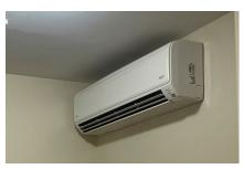
The home's air-source ductless mini-split heat pump has one outdoor variablespeed compressor and two indoor air handlers and provides very efficient heating and cooling (14 HSPF, 33 SEER).
