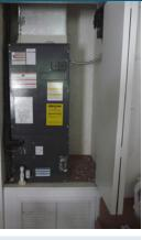
(left) The existing air handler was extremely leaky and mounted on a stand in the air handler closet. The closet was separated from the conditioned space by louvered doors, which restricted return air flow.
