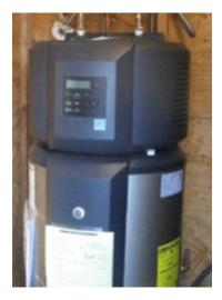
Installing a heat pump water heater in conditioned space can increase energy savings by reducing the load on space conditioning equipment. When there is insufficient room indoors for a heat pump water heater, which requires more clearance than a traditional electric resistance water heater, locating it in the attic or a connected space can also decrease cooling loads by cooling and dehumidifying the attic, the hottest part of the home in summer.
