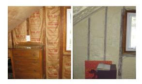
The side attics had a mixture of insulation types, including faced and unfaced fiberglass batt insulation *(left)*. These were replaced with closed-cell spray foam on the exterior walls and roof deck to provide a complete and continuous air barrier *(right)*, fully aligned with the vapor barrier. This reduced infiltration, mitigating the stack effect, which was pulling warm, moist air up into the attic.
