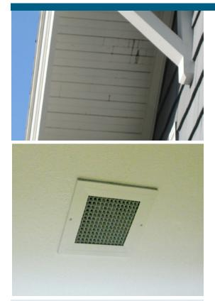
(*top*) Excessive humidity and condensation in the attic was causing unsightly staining and damage in the side attic spaces and on the eaves.
