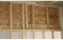
Many high performance improvements require attention to detail rather than a large investment. Electrical and plumbing holes were carefully sealed. Sill plate gasketing was used to seal sheetrock to the top plate. This is one of many low-cost improvements listed on the ENERGY STAR Thermal Bypass Checklist.
