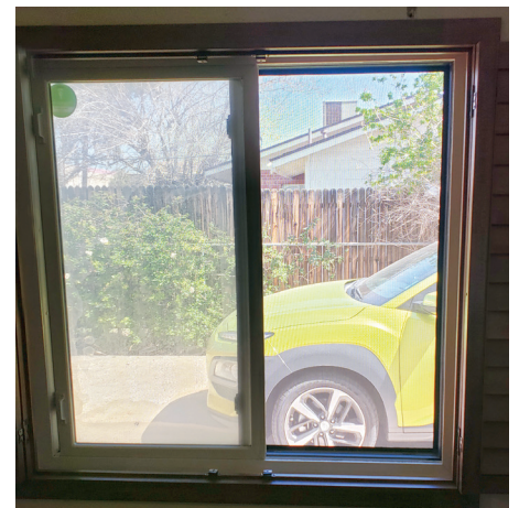
Solar screens were attached to the exterior of the window frames with Velcro-like attachments to reduce solar heat gain and views into the home while allowing views out.
