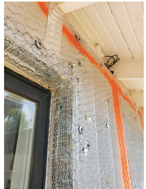
Stucco lath wraps around the windows and covers the 2 inches of foil-faced polyisocyanurate rigid foam that was installed over the original concrete block walls.
