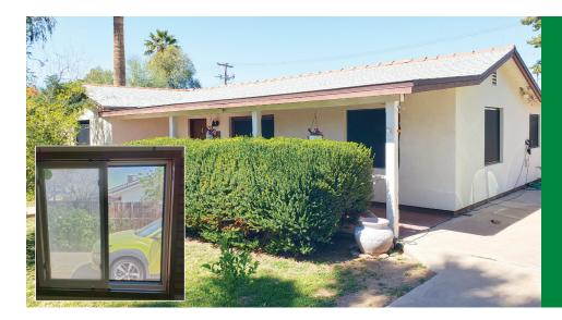
The original single-pane windows were replaced with double-pane low-e windows about 10 years ago. These double-pane windows remained but were upgraded with solar screens to reduce solar heat gain from the intense Arizona sun. Solar screens also provide privacy, limiting visibility into the home but providing visibility for those looking out. A unique hook and loop closure system keeps the screen in place without magnets or brackets.
