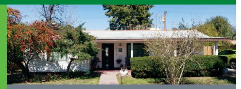
Rigid foam exterior insulation and solar screens were among the energy-saving retrofits to this 1950s concrete block home in Phoenix.
