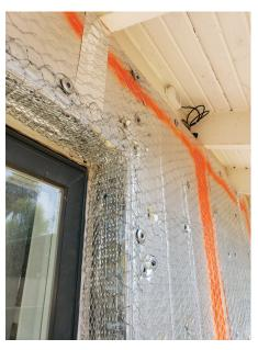
Stucco lath wraps around the windows and covers the 2 inches of foil-faced polyisocyanurate rigid foam that was installed over the original concrete block walls.
