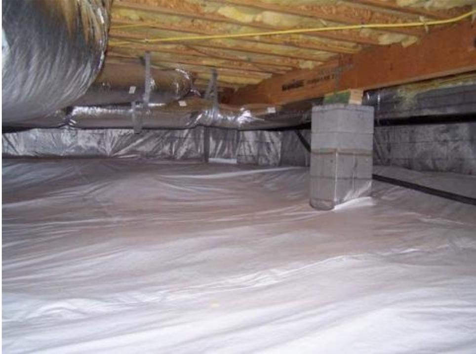
**Figure 2** - Polyethylene completely covers the floor of this crawlspace and is attached to the walls and piers as well to serve as a capillary break and continuous vapor barrier.
