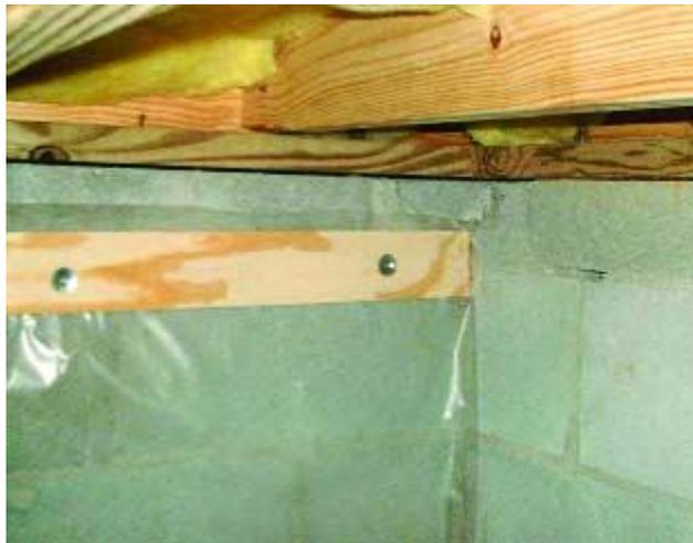
**Figure 3** - Polyethylene ground cover is attached to the crawlspace walls with plywood furring strips.
