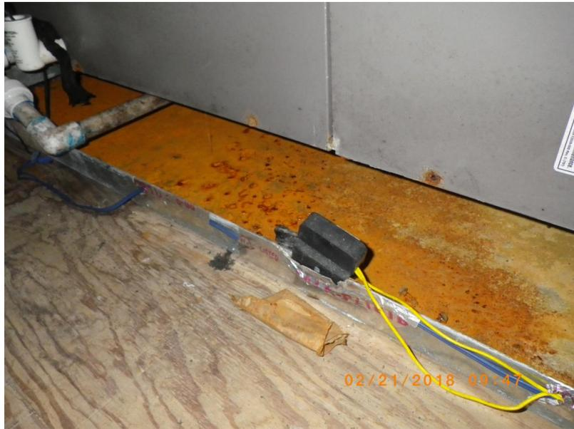
**Figure 3.** The HVAC equipment's condensate drain pan is equipped with a water-level detection device that will shut off the equipment if the water level in the pan gets too high. (Image courtesy of [Calcs-Plus](#))
