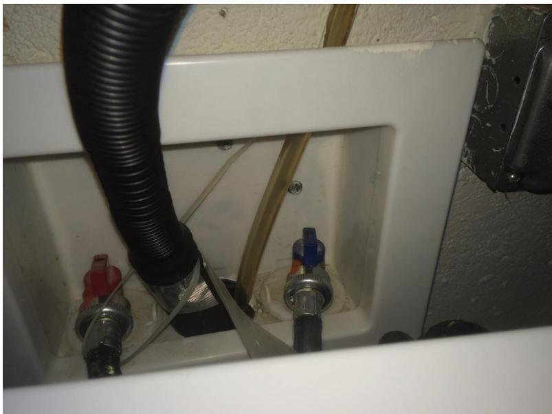
**Figure 6.** The condensate line (amber-colored plastic tube) from the high-efficiency furnace drains into the sewer via the same drain pipe as the clothes washer. (Image courtesy of Douglas Elliott, [PNNL](#))
