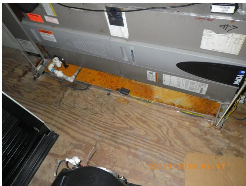
**Figure 2.** Metal drain pans under HVAC equipment can corrode over time, especially in humid environments. (Image courtesy of [Calcs-Plus](#))
