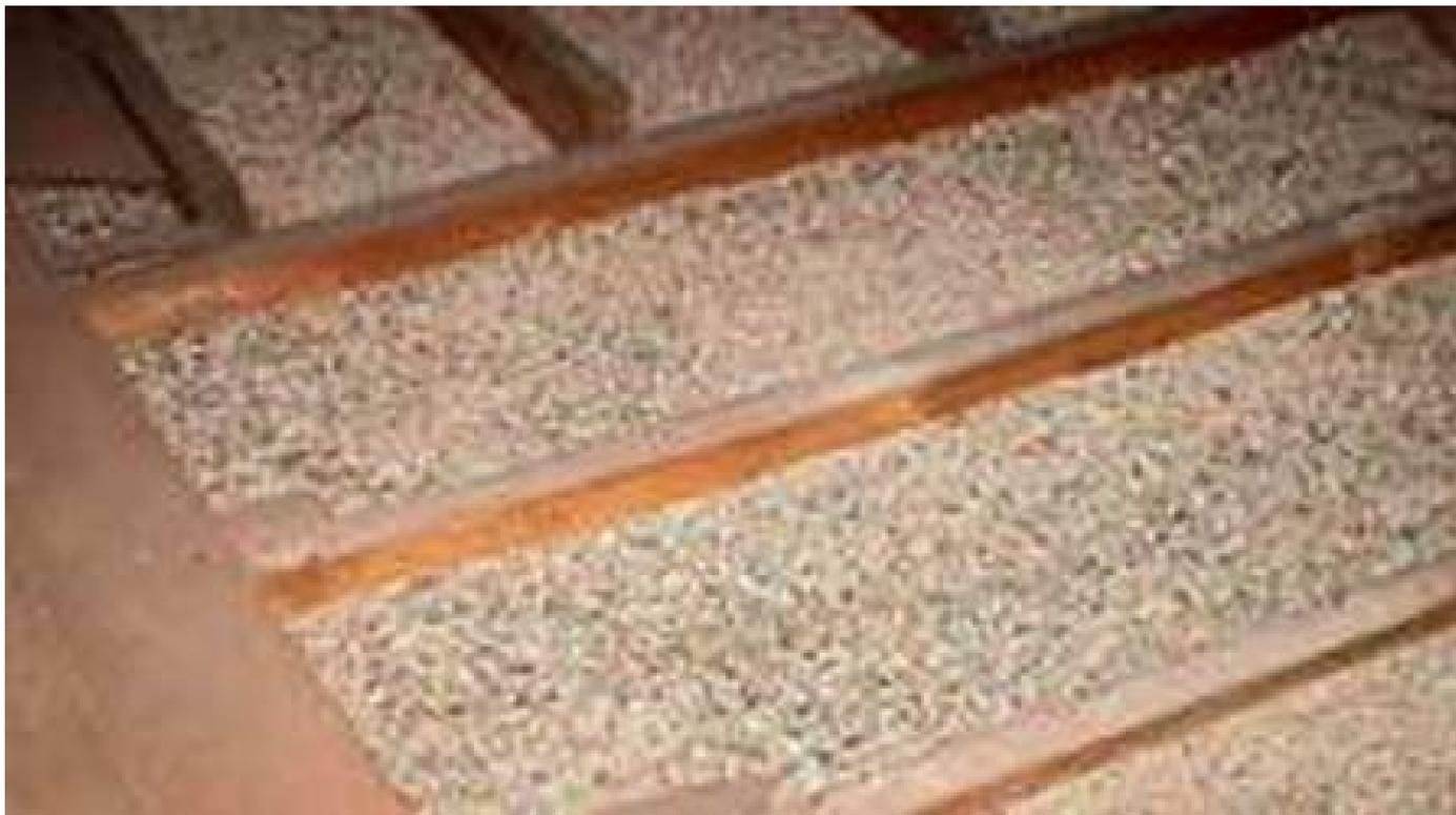
Vermiculite insulation between attic joists (image courtesy of [EPA](#) [2]).
