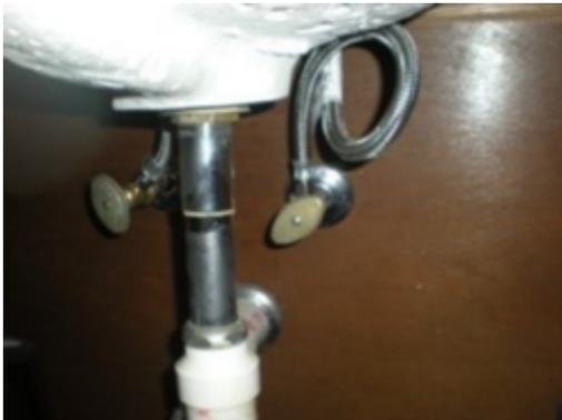
**Figure 2.** Plumbing leaks can occur in faucet fittings
