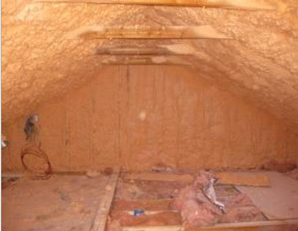
Insulate an attic in an existing home by installing spray foam (open cell or closed cell) on the underside of the roof deck. This measure will convert a vented attic to a nonvented attic. The installation steps are as follows:
