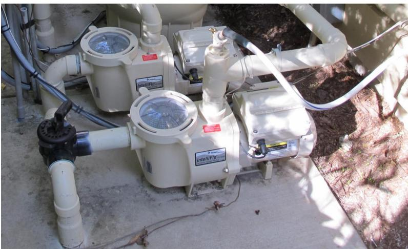
**Figure 2.** Variable-speed pool pumps can cut energy use by 50% to 90% compared to standard single-speed pumps (image courtesy of Steve Easley Associates).
