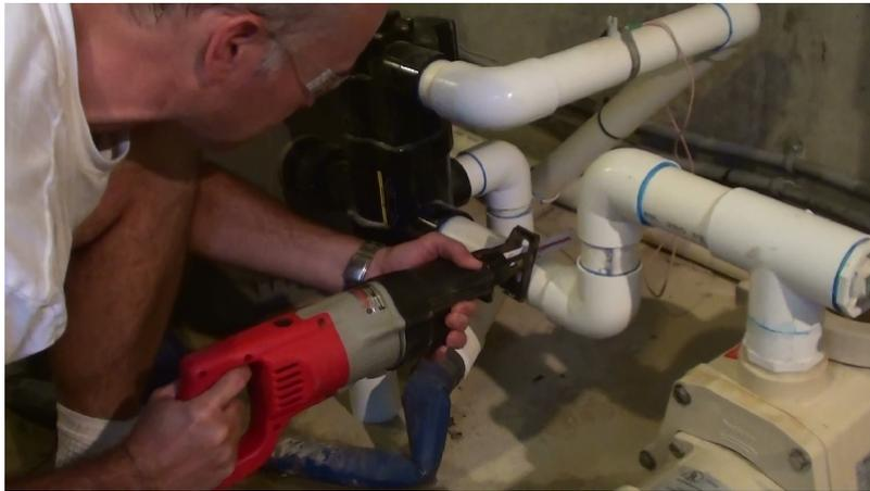
**Figure 3.** A reciprocating saw works well to cut PVC pipe during pool pump installation.
