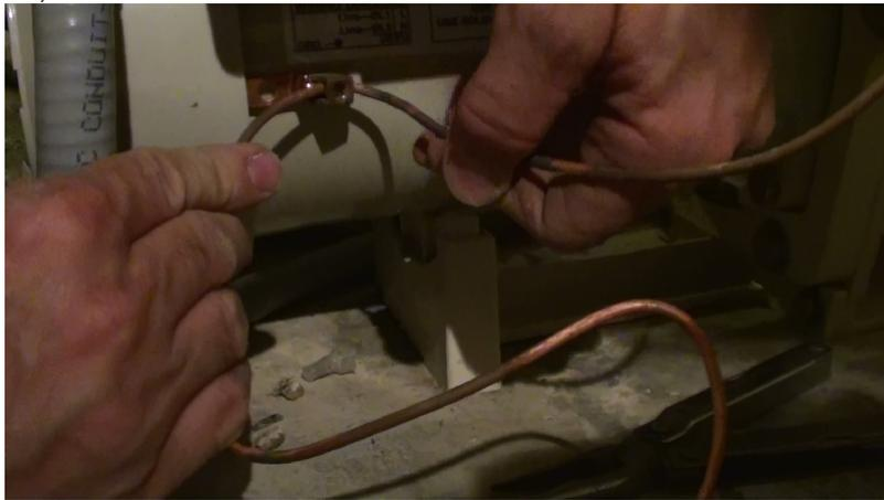
**Figure 4.** Make sure the ground bonding wire is securely fastened to the pump's bonding lug.
